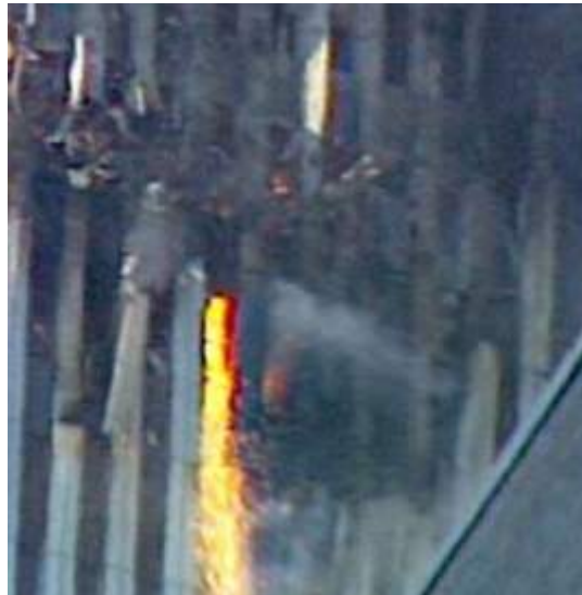
Molten metal pouring from Tower prior to collapse
