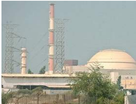
Iran's Bushehr Facility
