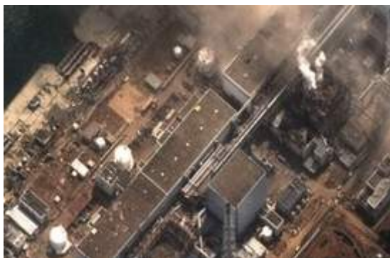
Steam appears from reactor 3 before explosion
